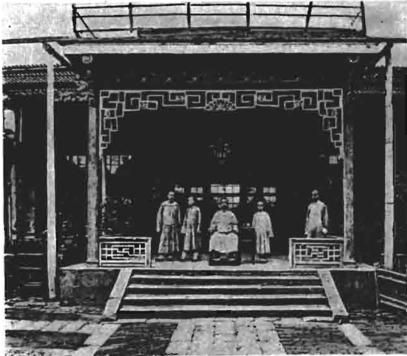
IV. 6—A COURT-HOUSE
